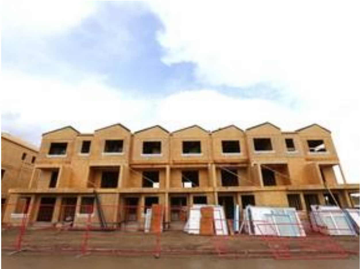
Townhomes under construction in East Hills Crossing in October. Jim Wells/Postmedia
