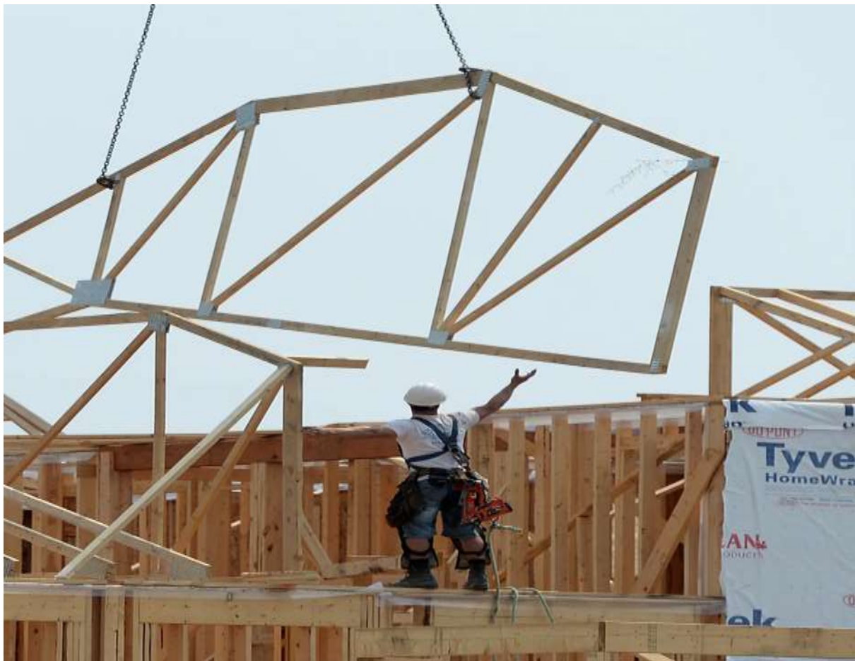
Construction workers build new homes in a development in Ottawa. Industry officials have largely applauded the federal government's new immigration targets, saying it's good for business. (Sean Kilpatrick/The Canadian Press)
