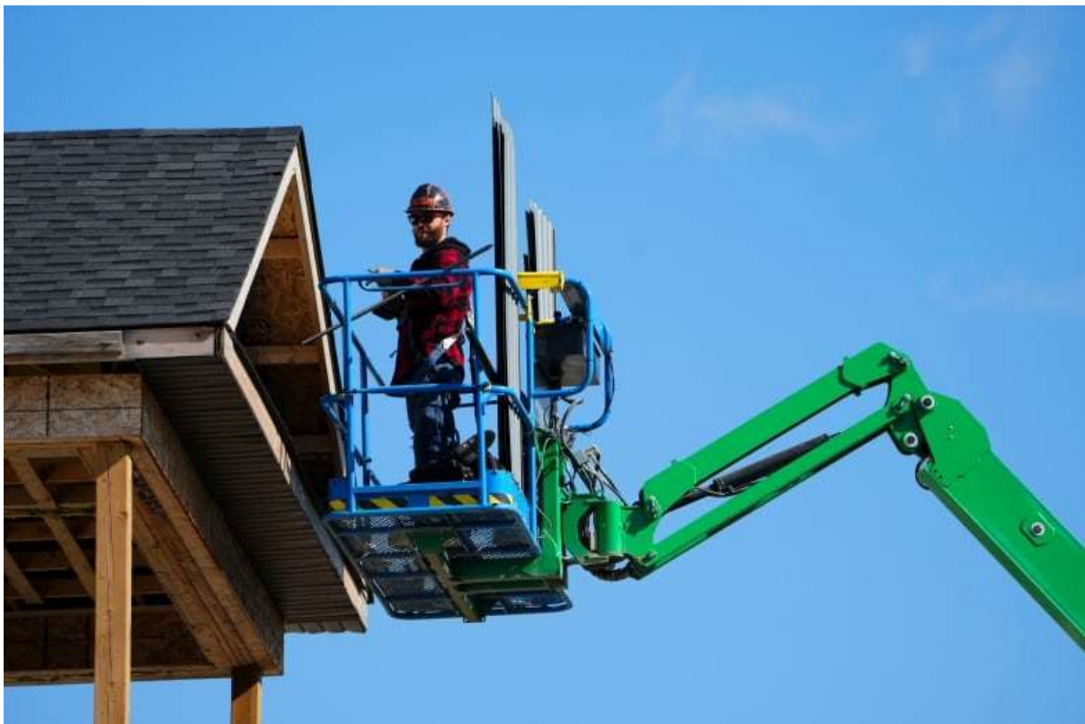
A construction worker stands on a lift in a new housing development in Ottawa in October. An influx of new citizens is more likely to affect rents than house prices, according to data experts. (Sean Kilpatrick/The Canadian Press)
